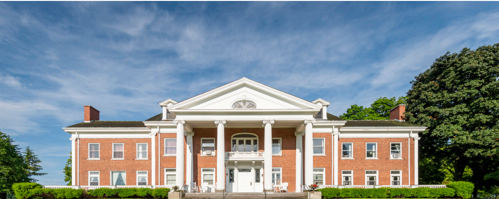
White Springs Manor Located two miles west of Belhurst Castle
